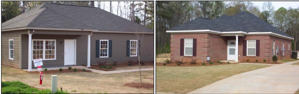
Houses in the Northwest Village Subdivision
