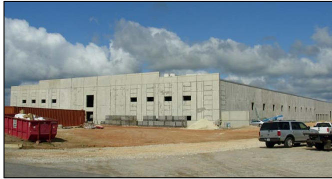
Construction of Sio2 Medical Products Inc. Facility in Auburn
